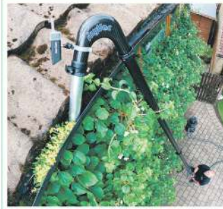
Gutter Cleaning with SkyVac
