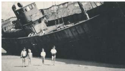
S T Sheraton c 1948 – a dangerous playground
