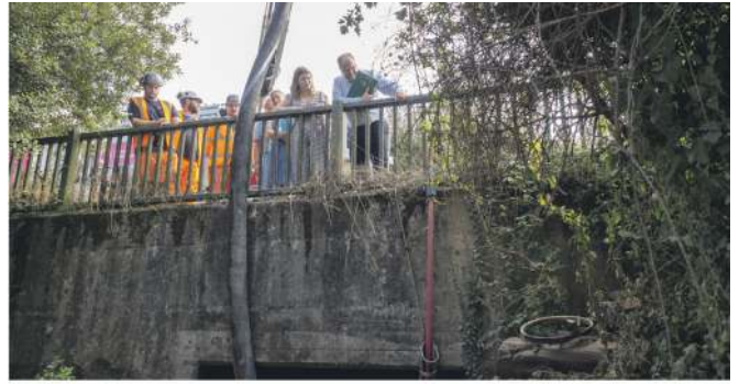
Flood Alliance partners undertake major clear-up operation in Attleborough, 2024. Picture Credit: Norfolk County Council
