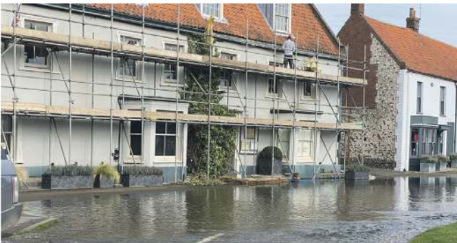
Flooding in Burnham Market, 2021
