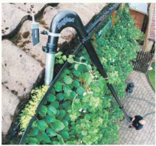
Gutter Cleaning with SkyVac
