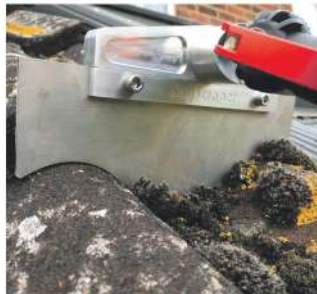
Moss Removal with Skyscraper
