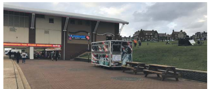
The Hangar viewed from the south in August 2021
