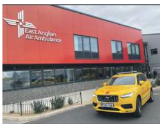
EAAA Helimed House Norwich Airport
