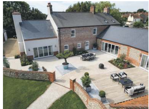
GR Coastal Groundworks project
