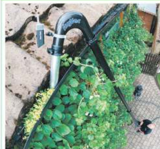
Gutter Clearing with SkyVac
