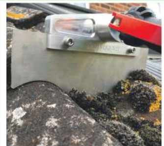
Moss Removal with Skyscraper
