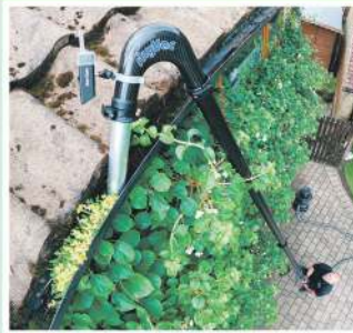
Gutter Cleaning with SkyVac
