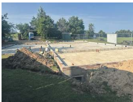
Thornham Clubhouse progress
