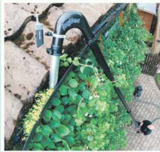
Gutter Cleaning with SkyVac
