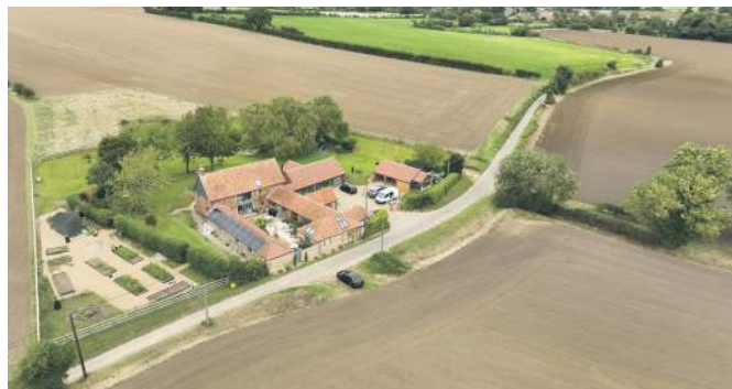
Aerial view of the finished scheme
