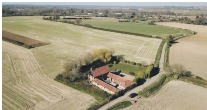
Aerial view of the existing site before the project
