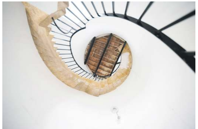
The spiral staircase in the lighthouse
