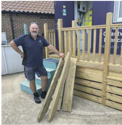
New platform decking
