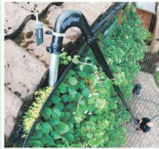
Gutter Cleaning with SkyVac
